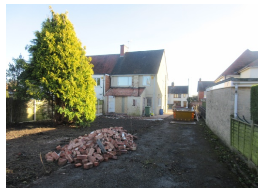
Photo taken facing east towards No 68 Storrs Road
